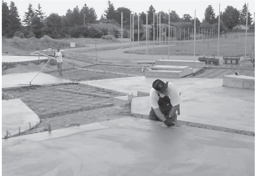
Visitors need to respect the "Keep Out" signs to avoid damaging the new concrete and causing further delays for repairs.
