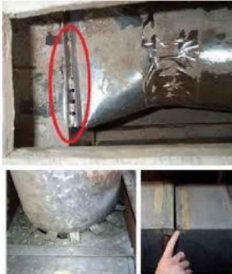
This code recognizes that successful achievement of State energy use reduction goals cannot solely depend on new construction requirements. Research has found that a lot of energy is consumed heating air that leaks from ducts located in unconditioned spaces such as crawlspaces and attics. unconditioned space can lose 15 to 30% of your heated before it even gets to the register. Not only is this an avoidable waste of energy; it costs homeowners a lot of money since you are heating the outside!
